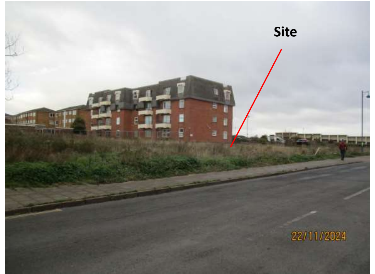
From east side
