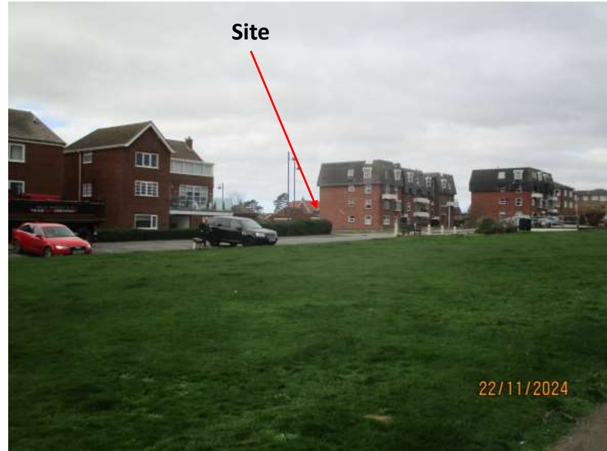
Southwest adjacent to play area
